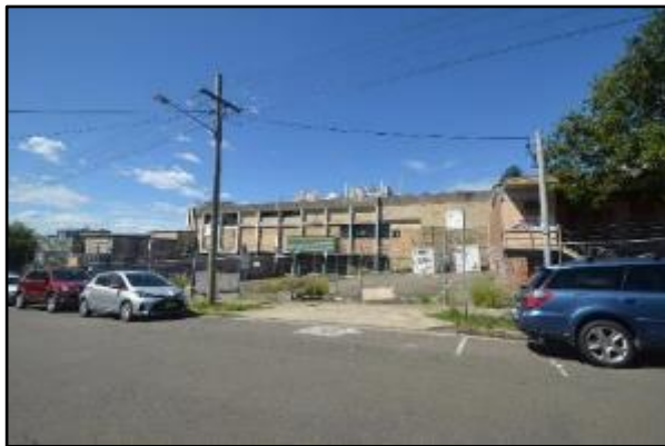
Figure 39. View of the of the Balmain Leagues Club from Waterloo Street (Source: Heritage 21, 15.01.18)
