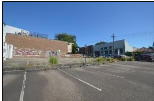
Figure 42. The Boundary wall constructed across 1 Waterloo Street visible from parking lots on 3 – 7 Waterloo Street (Source: Heritage 21, 15.01.18)
