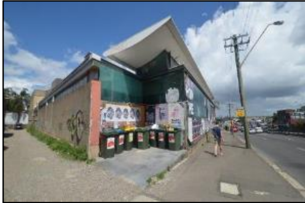
Figure 31. View of The Balmain Leagues Club boundary along the rear alleyway of the Darling Street Properties (Source: Heritage 21, 30.11.17)
