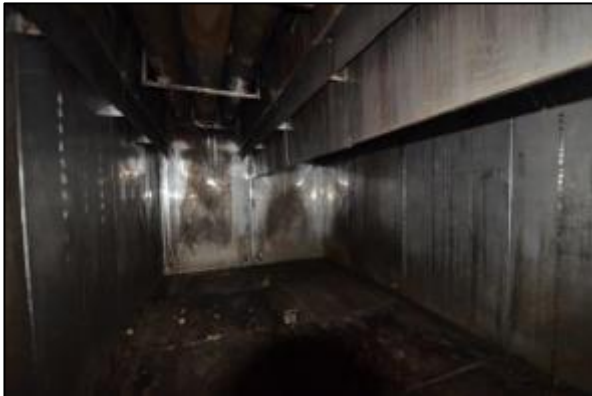
Figure 63. Cold Storage rooms in butcher shop on 699 Darling Street (Source: Heritage 21, 15.01.18)
