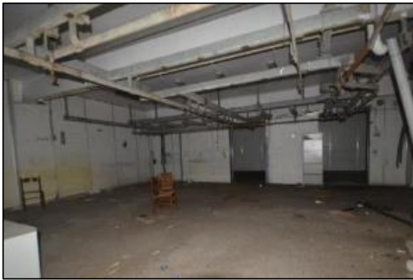
Figure 61. Interior view of butcher shop on 1 Waterloo Street (Source: Heritage 21, 15.01.18)
