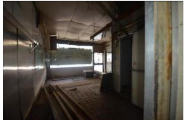
Figure 64. Shop front view from interior, 699 Darling Street (Source: Heritage 21, 15.01.18)
