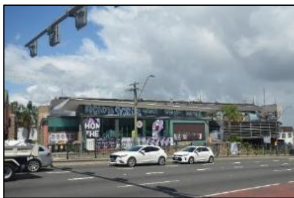
Figure 30. View of Balmain Leagues Club Building from Victoria Road (Source: Heritage 21, 30.11.17)
