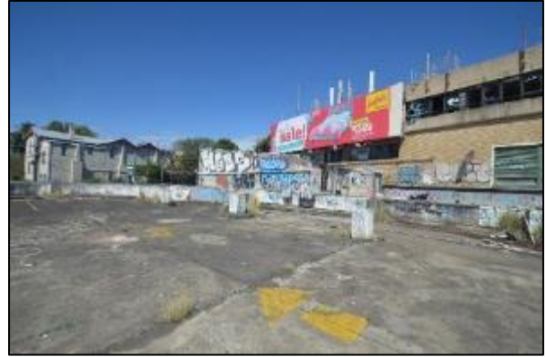
Figure 44. View of the main club building from the upper level parking lot (Source: Heritage 21, 15.01.18)
