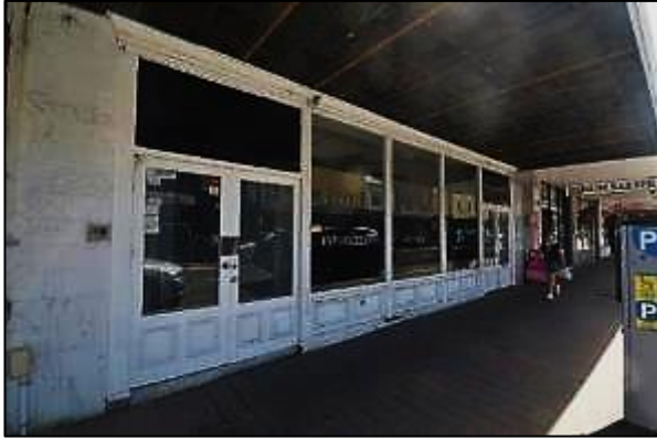
Figure 47. Ground floor entrance to the Byer's Building on 697 Darling Street (Source: Heritage 21, 30.11.17)
