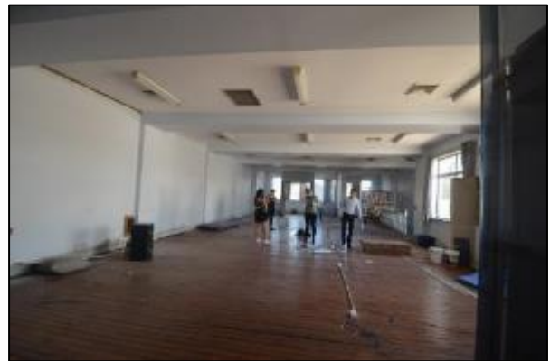
Figure 56. View of the main hall on the first floor, 697 Darling Street (Source: Heritage 21, 30.11.17)
