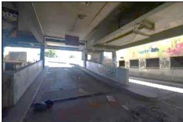
Figure 47. View of ramp to Upper Level car park (Source: Heritage 21, 15.01.18)
