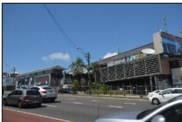
Figure 29. View of Balmain Leagues Club Building from Victoria Road (Source: Heritage 21, 30.11.17)
