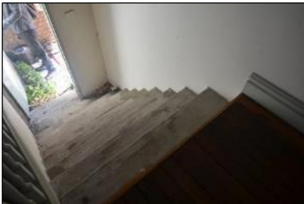
Figure 51. Stairs leading to rear alley on Darling street (Source: Heritage 21, 30.11.17)
