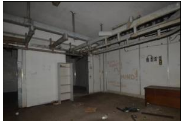
Figure 62. Interior view of butcher shop on 1 Waterloo Street (Source: Heritage 21, 15.01.18)
