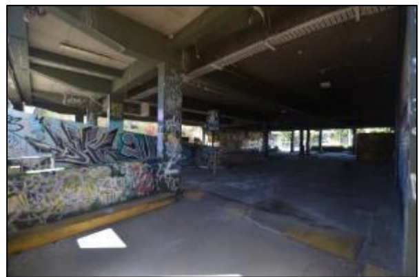
Figure 46. View of Ground Level car park (Source: Heritage 21, 15.01.18)
